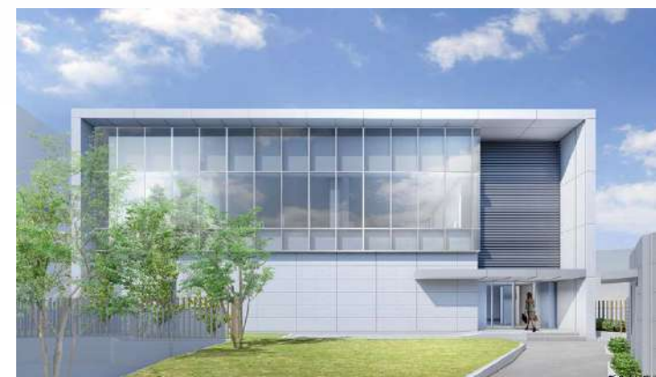
New Synthesis Research Wing (under construction)
